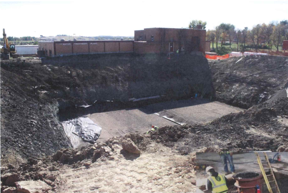
Construction of the Finished Water Pump Station
